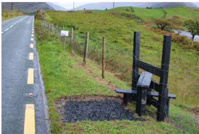
New stiles made from aluminium (top) and recycled plastic (bottom).
